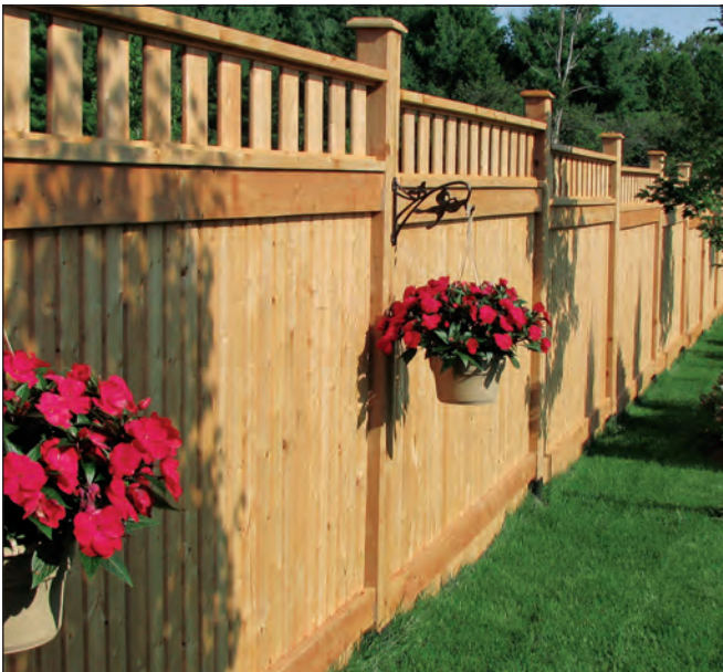
Micronized iron oxide pigments added to the wood preservative gives colour to pressure-treated wood.
