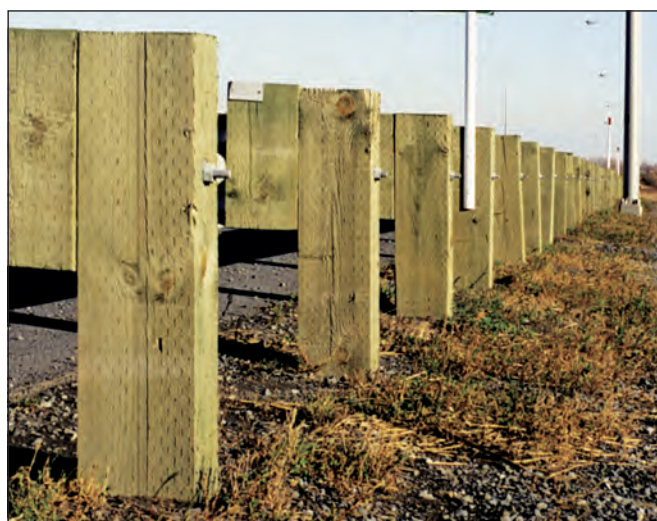
Chromated copper arsenate (CCA) continues to be used in industrial and non-residential applications, such as highway guardrails.
