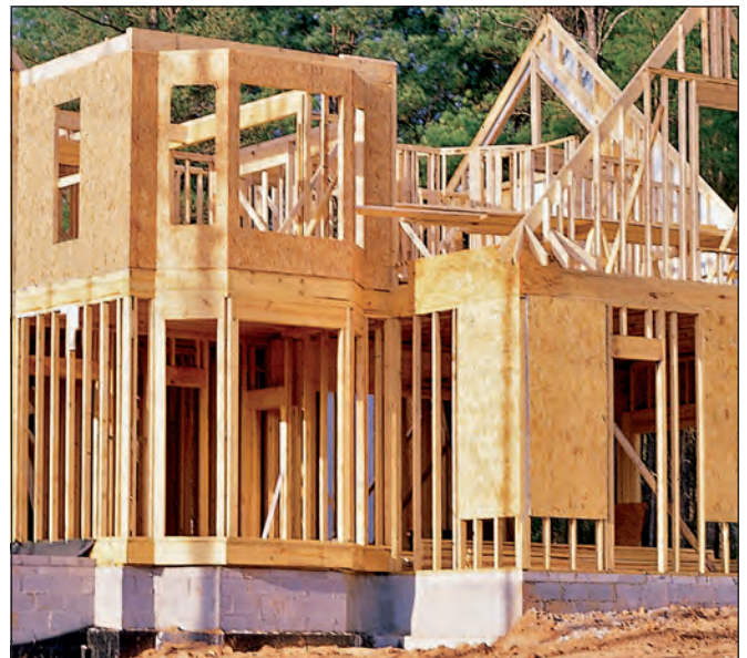
Borate pressure treatment protects lumber and plywood products used in protected or interior construction.
