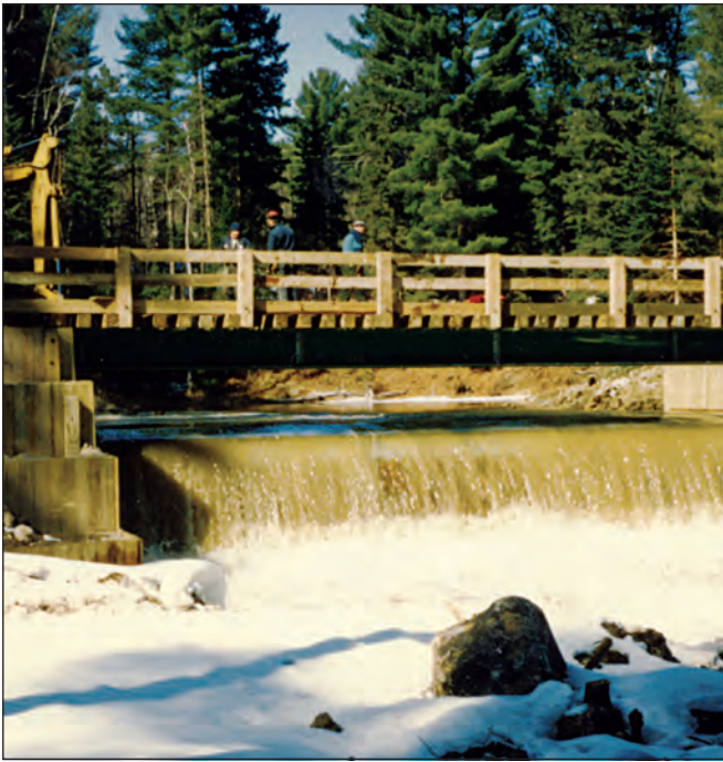
Pentachlorophenol (PCP)-treated timbers have commonly been specified for wood bridge construction.
