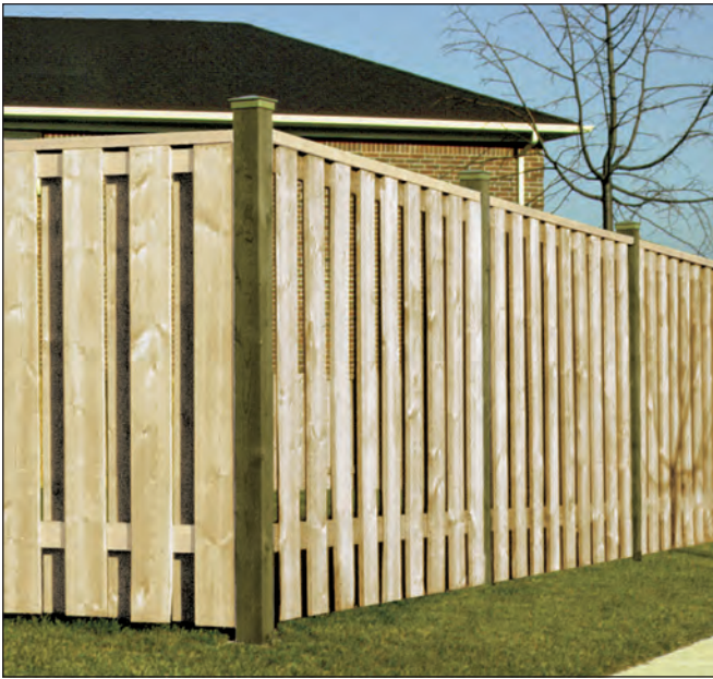
Carbon-based wood preservatives are colourless. This allows the natural appearance of 'ordinary' wood to be maintained.
