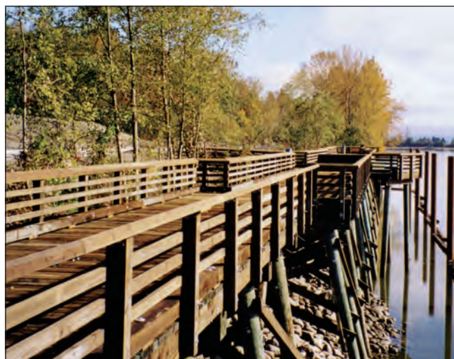
Creosote-treated marine pilings support a waterside pedestrian walkway.
