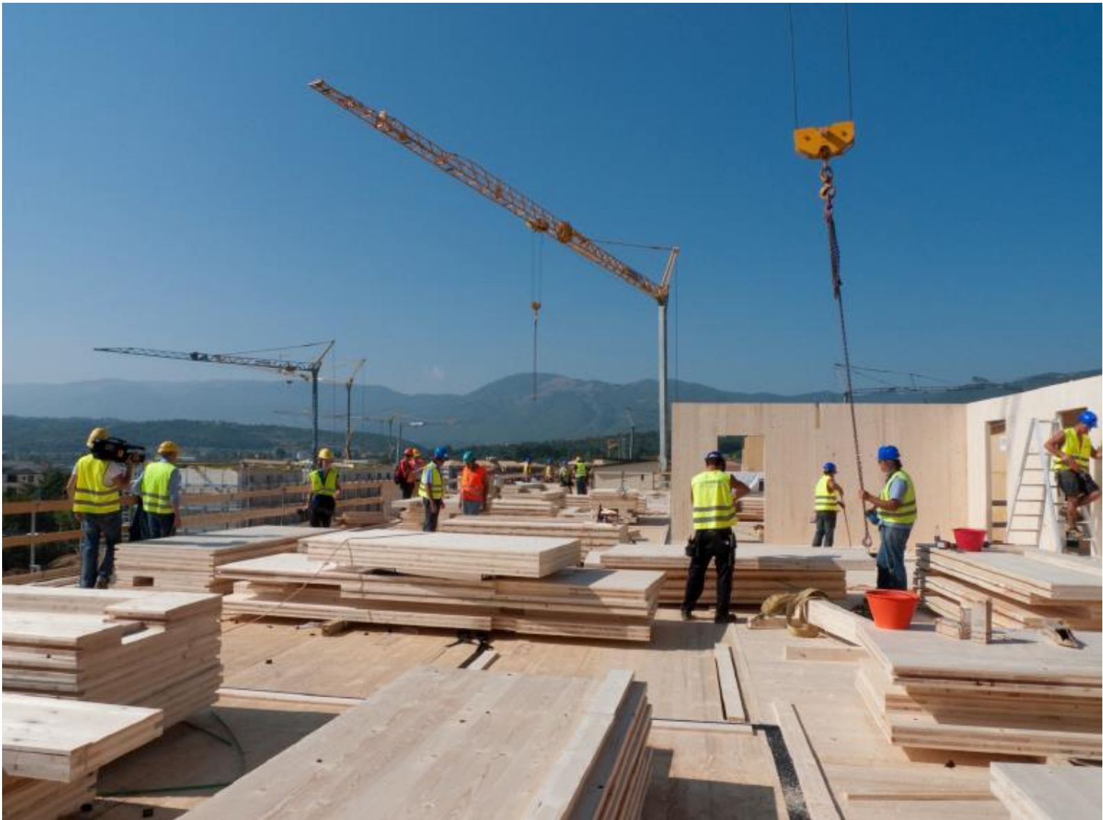
Italy – Multi-storey CLT project (Source: promolegno - proHolz)
