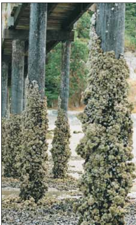
The personal use pier shown here is constructed of creosote-treated piling with ACZA-treated walkways
