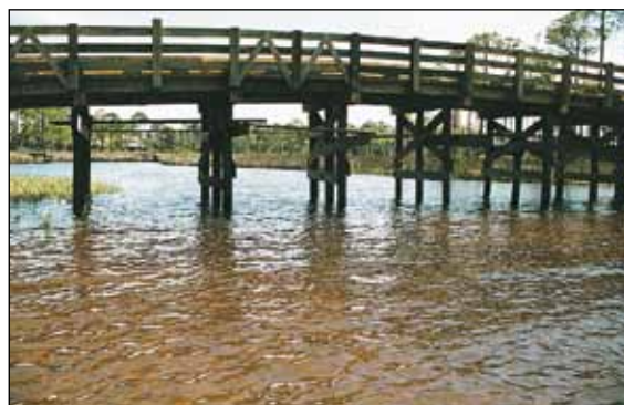
Horseshoe Bayou Bridge
