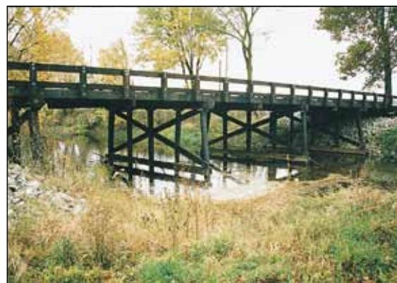
Pipe Creek Bridge
